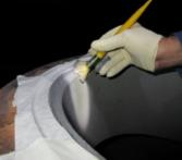
High temperature vessel suffering from severe corrosion. Pitted surface rebuilt using with Belzona 1511.
